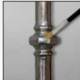
Application of the passivating product E4052/P: the polluted component must entirely be covered
