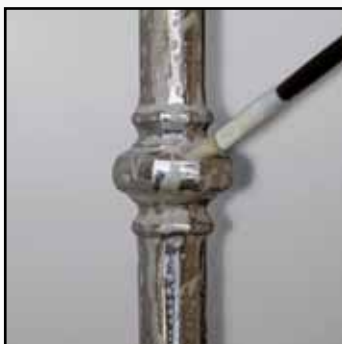
Applicazione del derugginante E4052/D deve coprire tutte le parti inquinate Application of the de-rusting product E4052/D: all polluted parts must be covered
